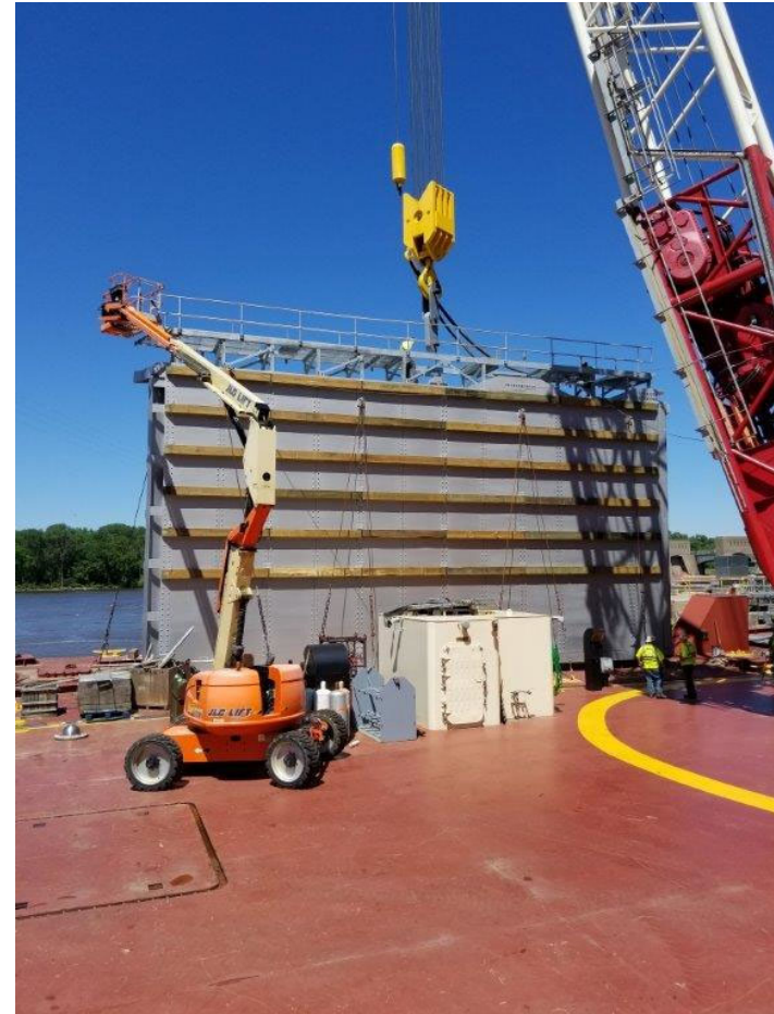
Left to Right: Removing an old miter gate (LD8); Preparing to pick a new miter gate for placement (LD8).
